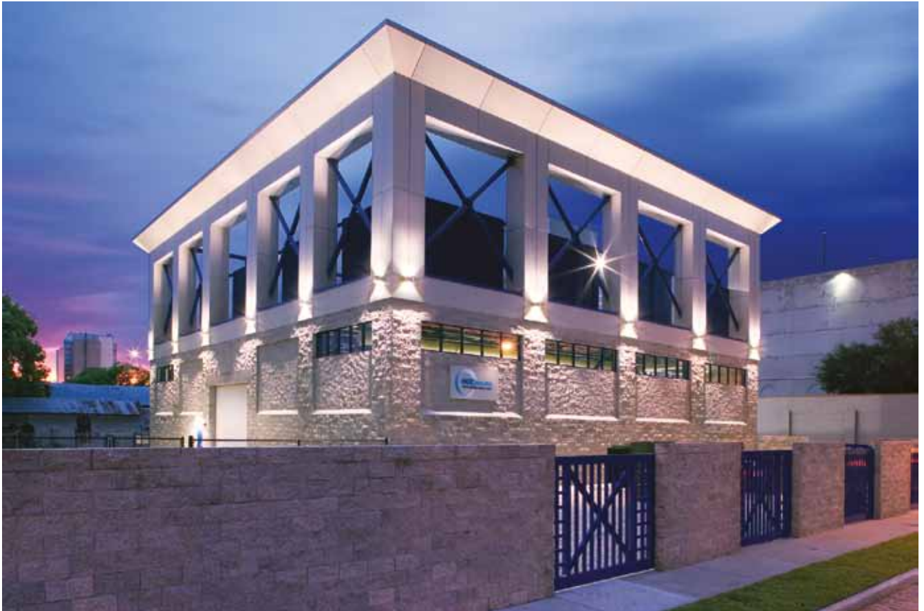
Figure 26: Municipally-owned OUCooling provides innovative, reliable cooling to customers in downtown Orlando Image courtesy of Orlando Utilities Commission.
