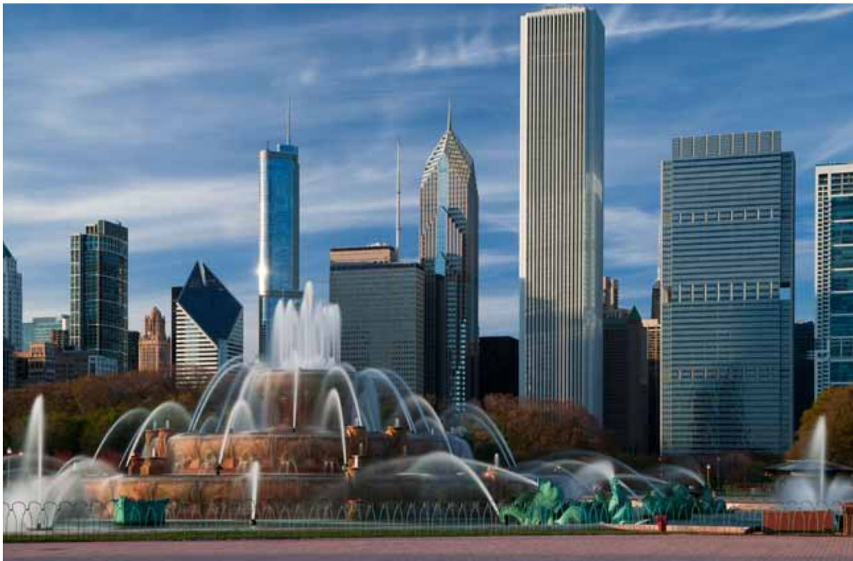
Figure 24: District energy will provide clean, cost-effective energy services to a brownfield site in South Chicago.
