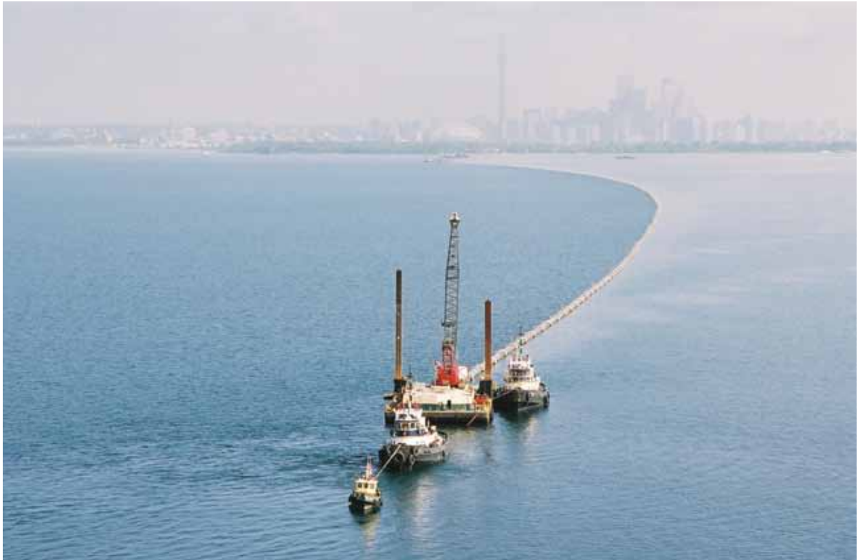
Figure 17: Enwave's Deep Lake Water Cooling uses the icy water of Lake Ontario to provide renewable cooling for the city of Toronto.
