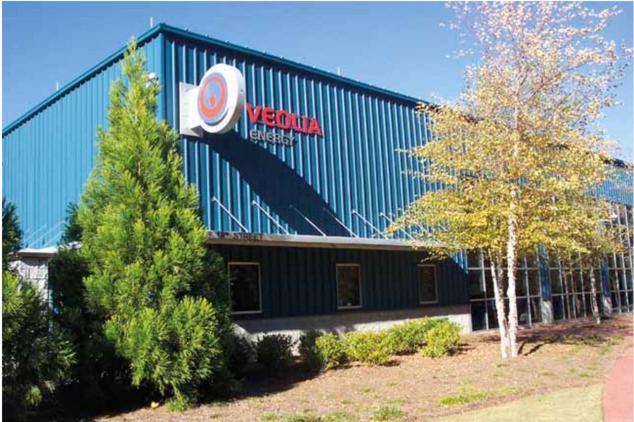
Figure 21: A central chilled water plant and district cooling network provide efficient air conditioning to the buildings in Atlantic Station, a model mixed-use development in Georgia
