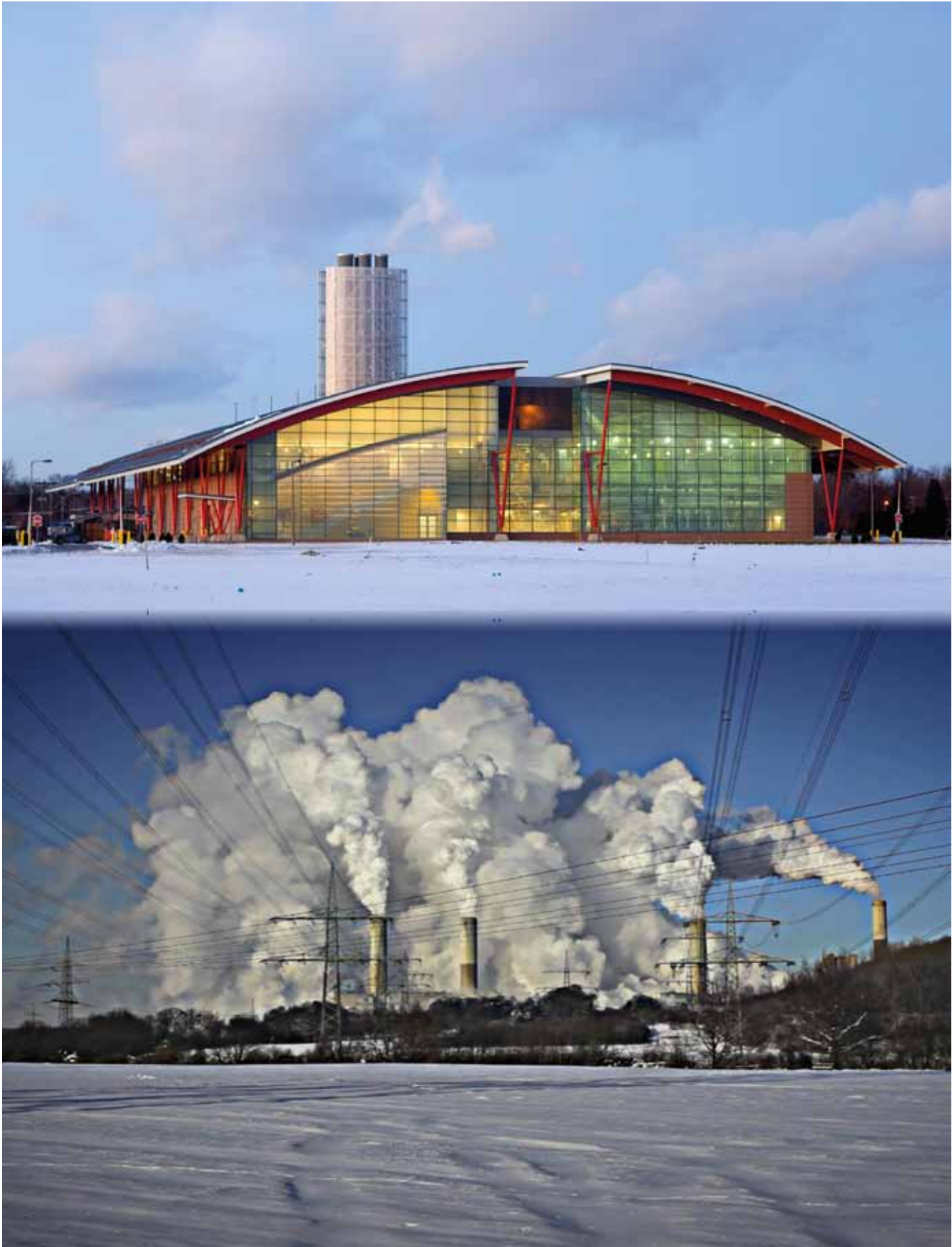
Figure 4: Institutions such as the University of Massachusetts, Amherst operate highly efficient district energy and CHP systems (top picture) to capture and use the heat that is wasted by typical central power generation (bottom picture).
